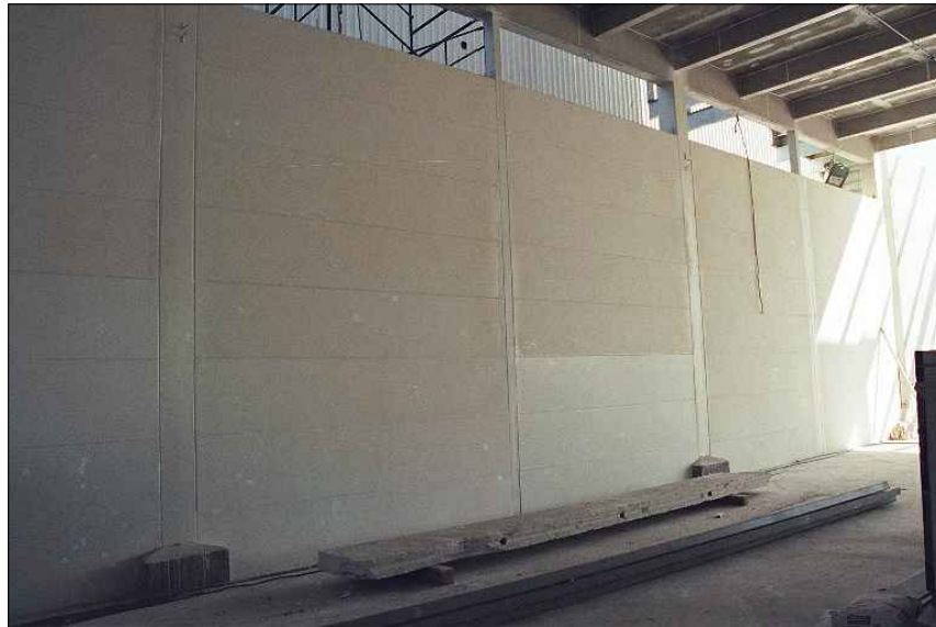
VISTA INTERIOR DE PANEL MURO HEBEL
